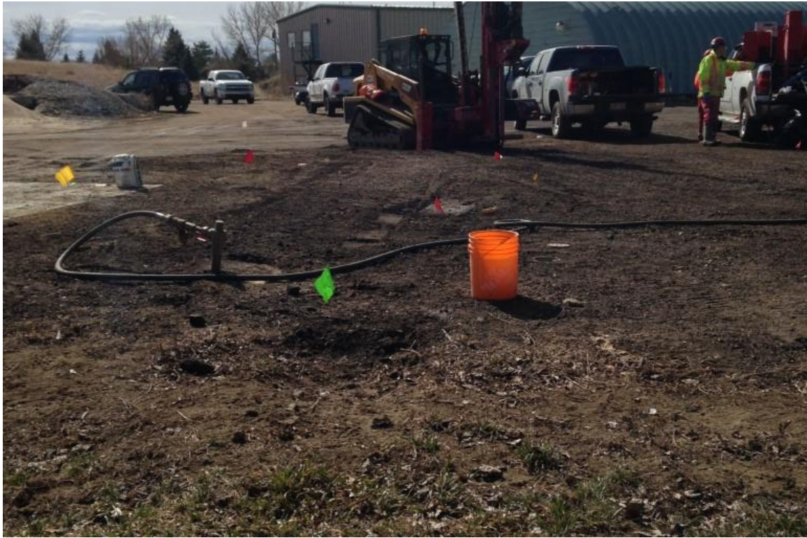
In-Situ Chemical Injection of contaminated area
