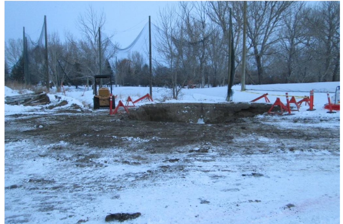
Second, larger excavation of impacted area
