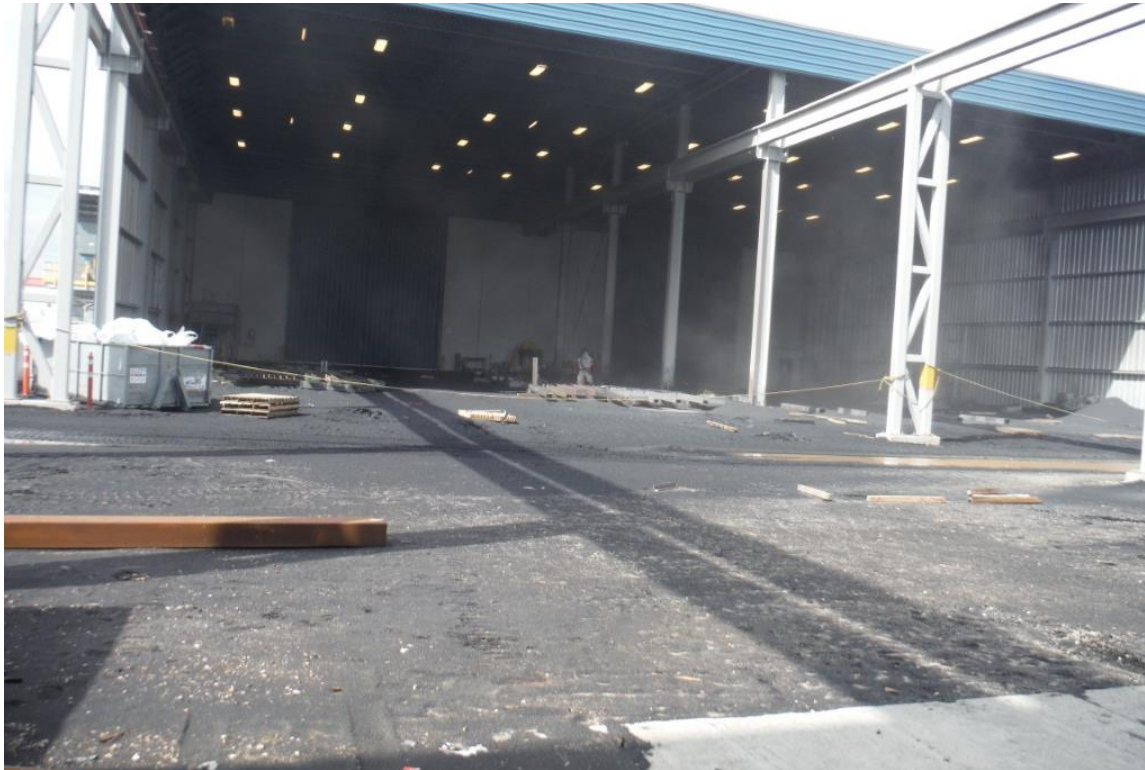
View of partially covered sand blasting area
