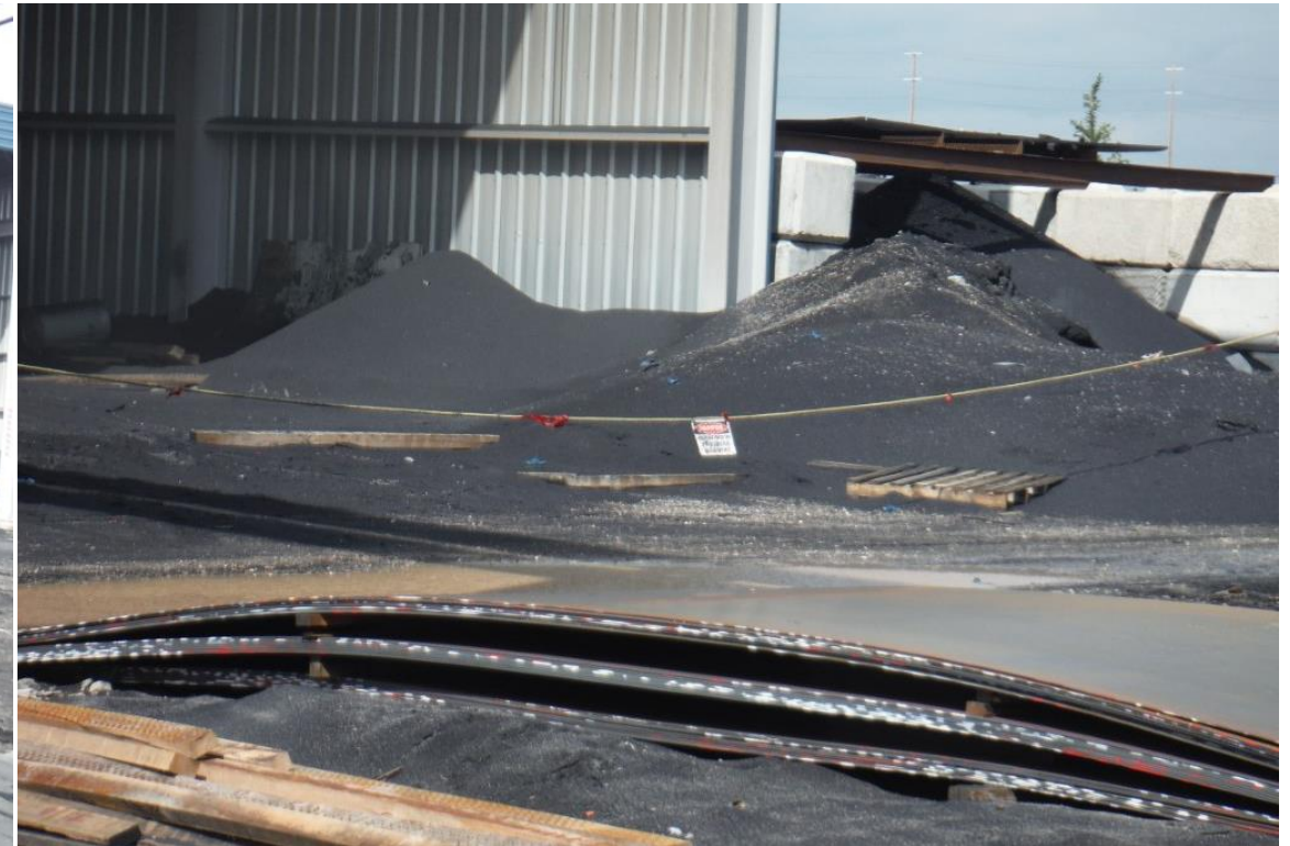
View of stored sand placed beyond the limits of the covered storage yard
