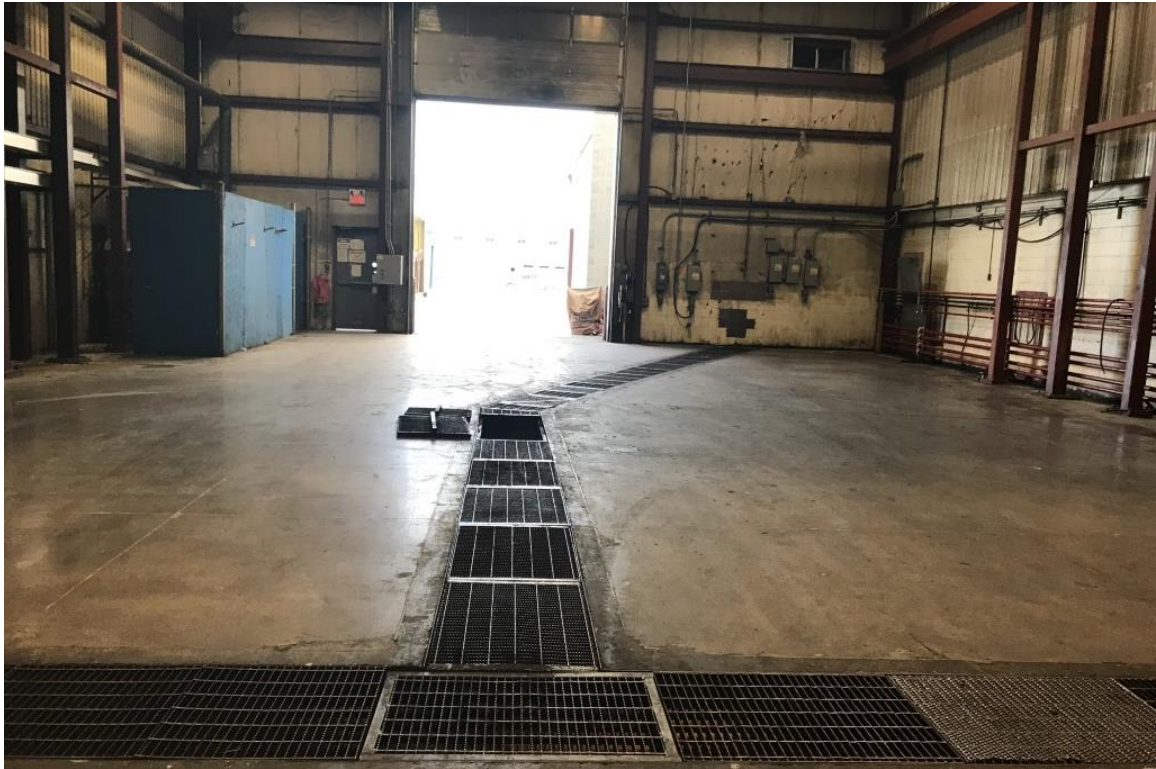
View of the damaged OWS and drain lines prior to excavation
