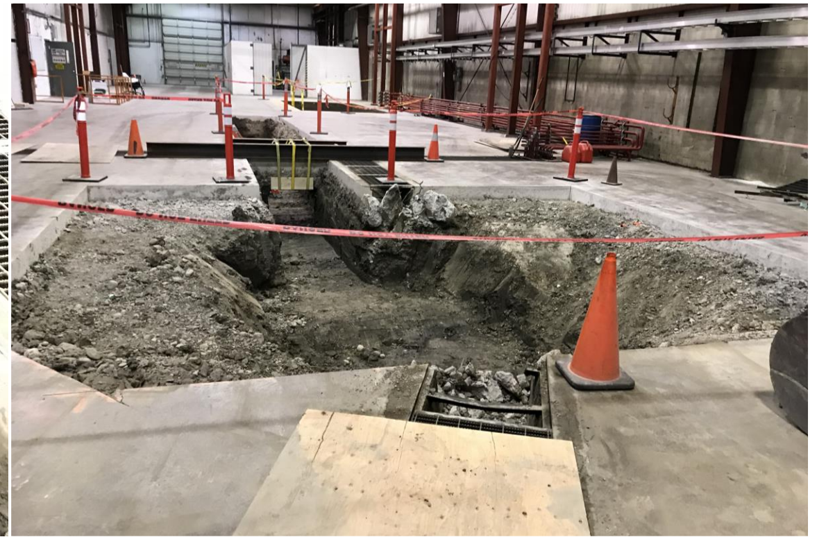
View of excavation around former OWS separator
