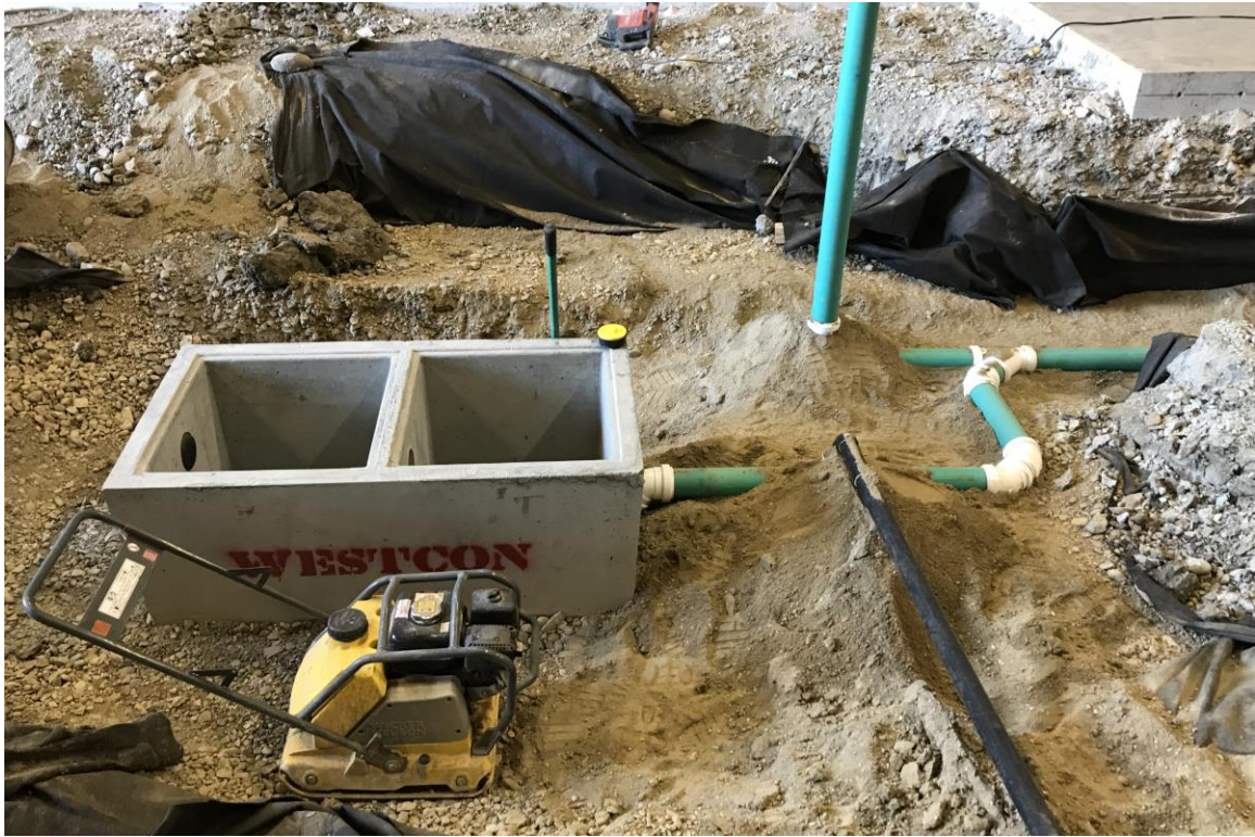
View of newly installed OWS system
