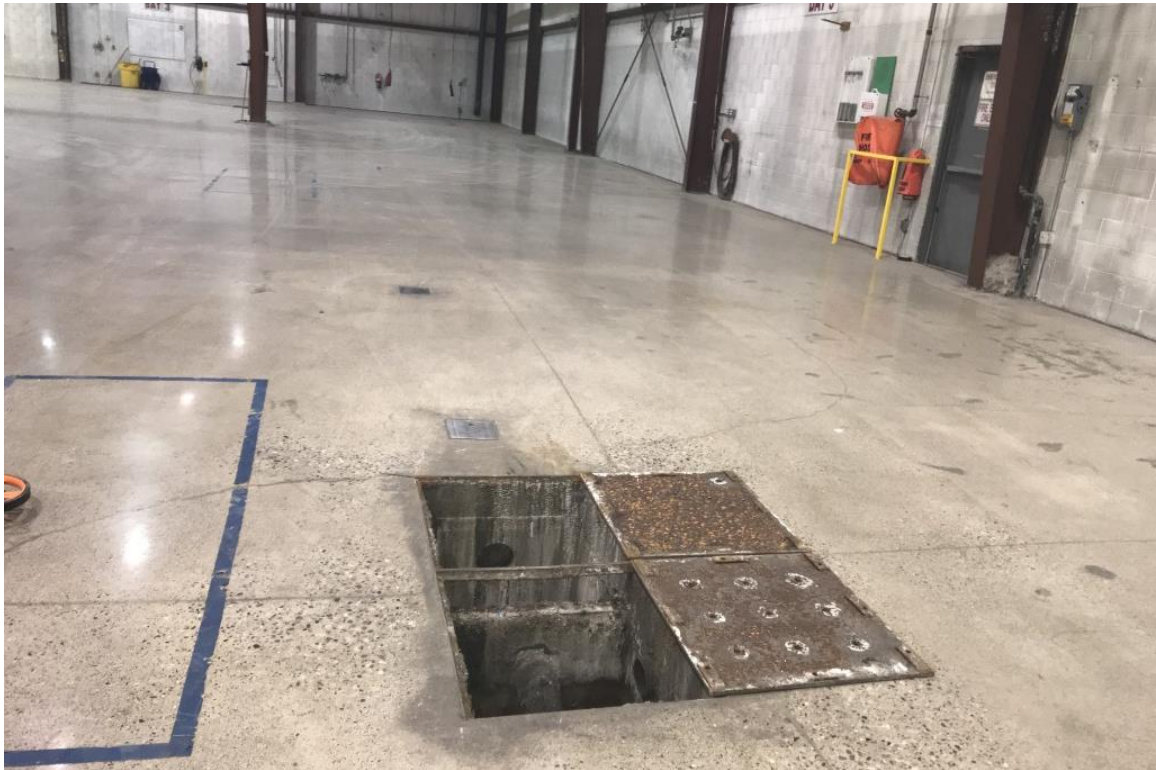
View of a typical dual-staged oil/water separator (OWS)
