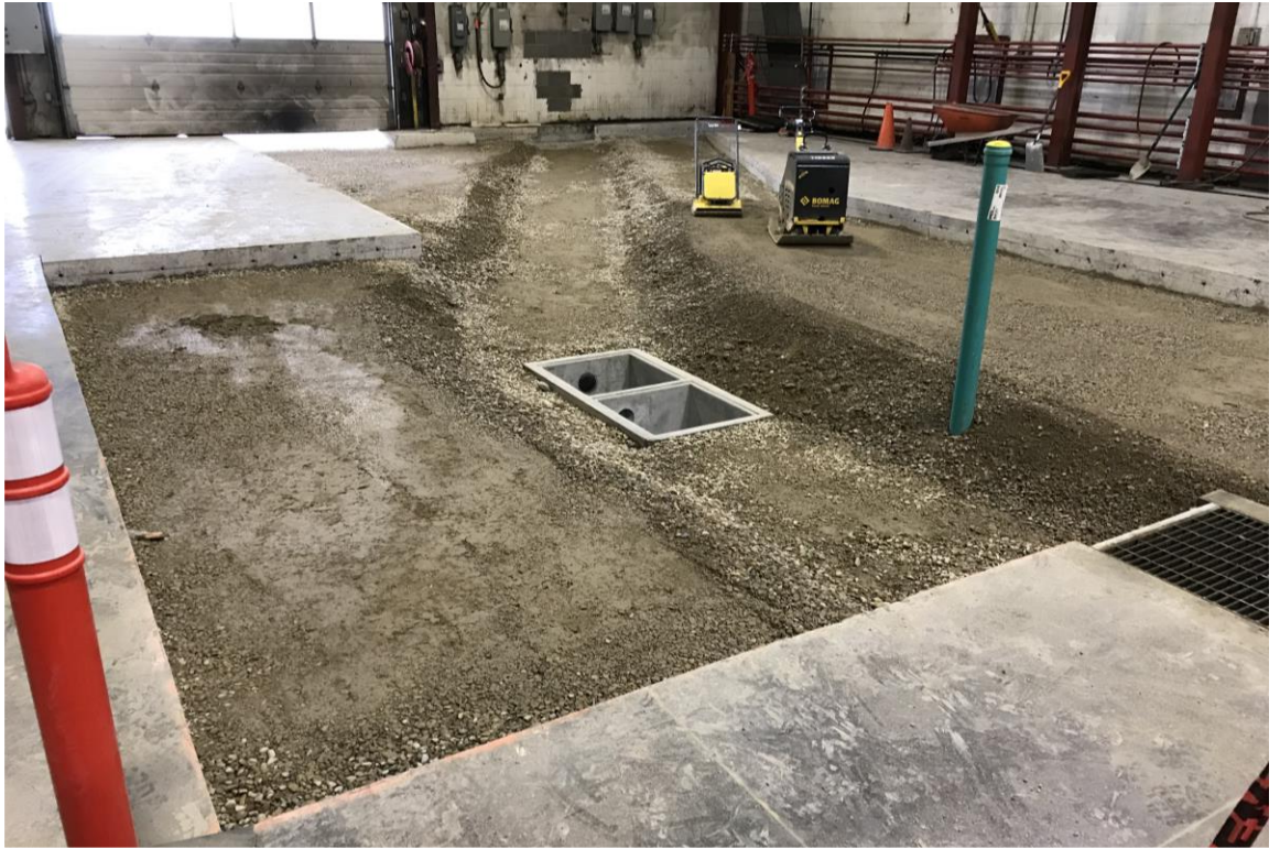
View of a portion of the excavation
