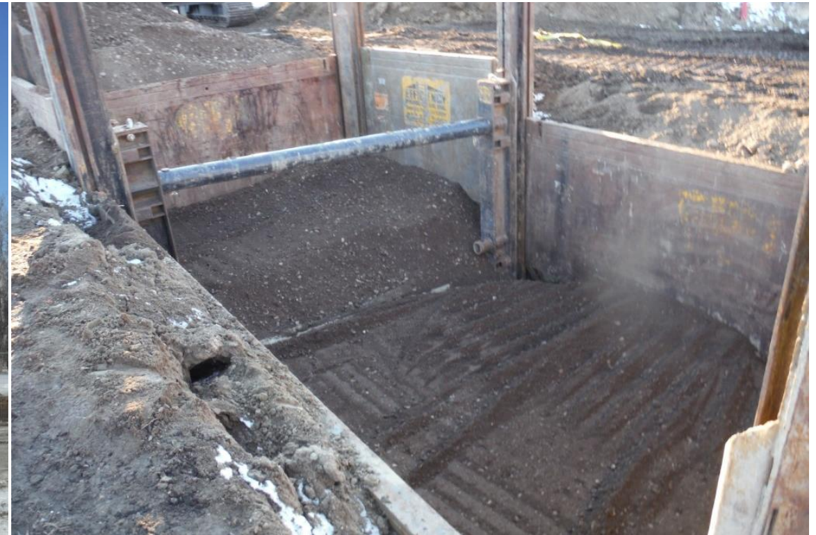
Fourth Excavation with more slide rail shoring
