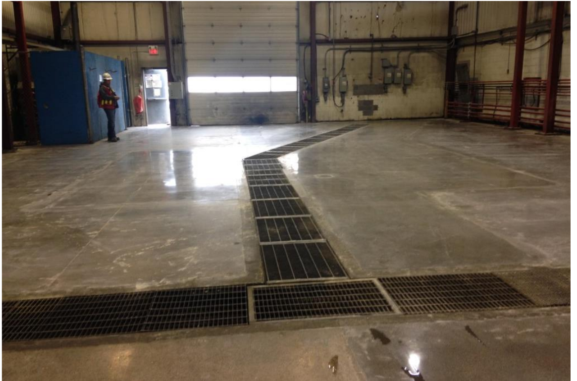
View of the newly installed OWS and drain lines post excavation
