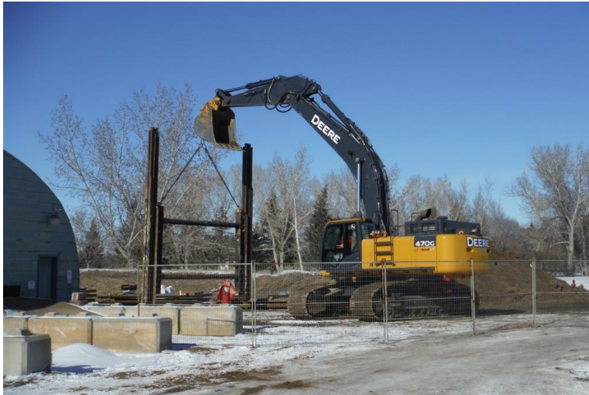
Third round of excavating with the installation of slide rail shoring
