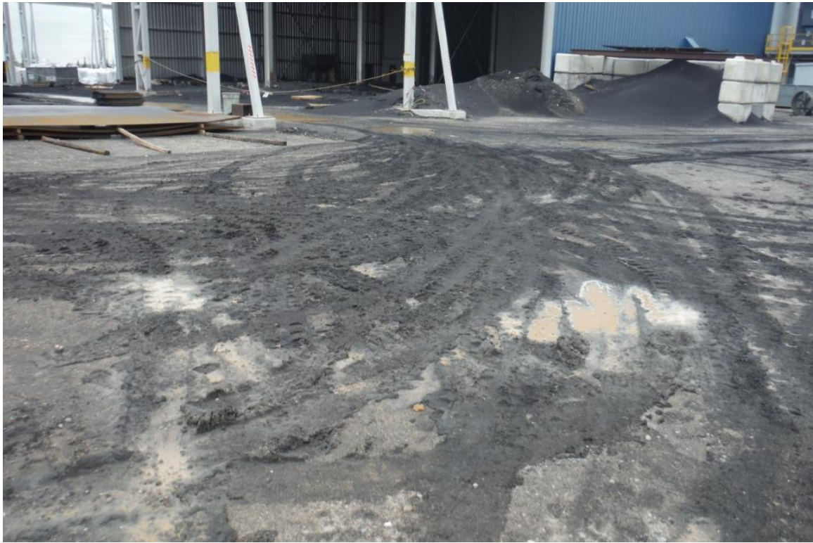
General view of spent sand observed throughout the storage yard
