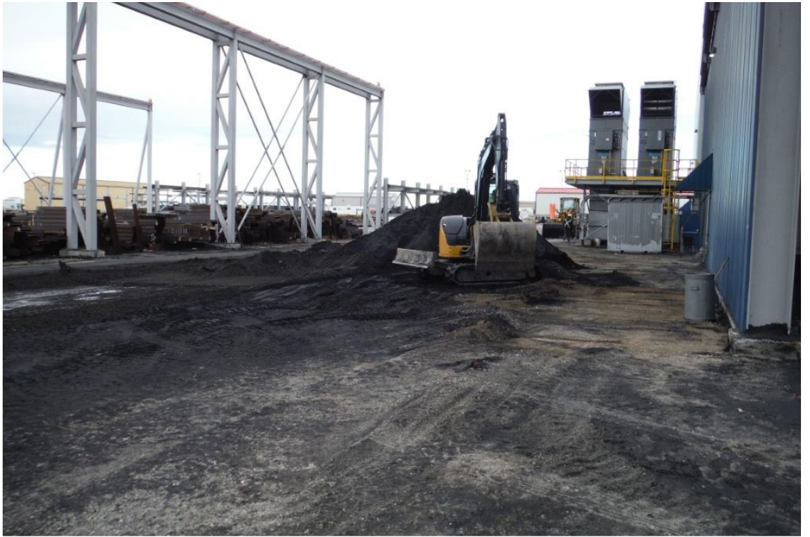
View of excavation of spent sand material
