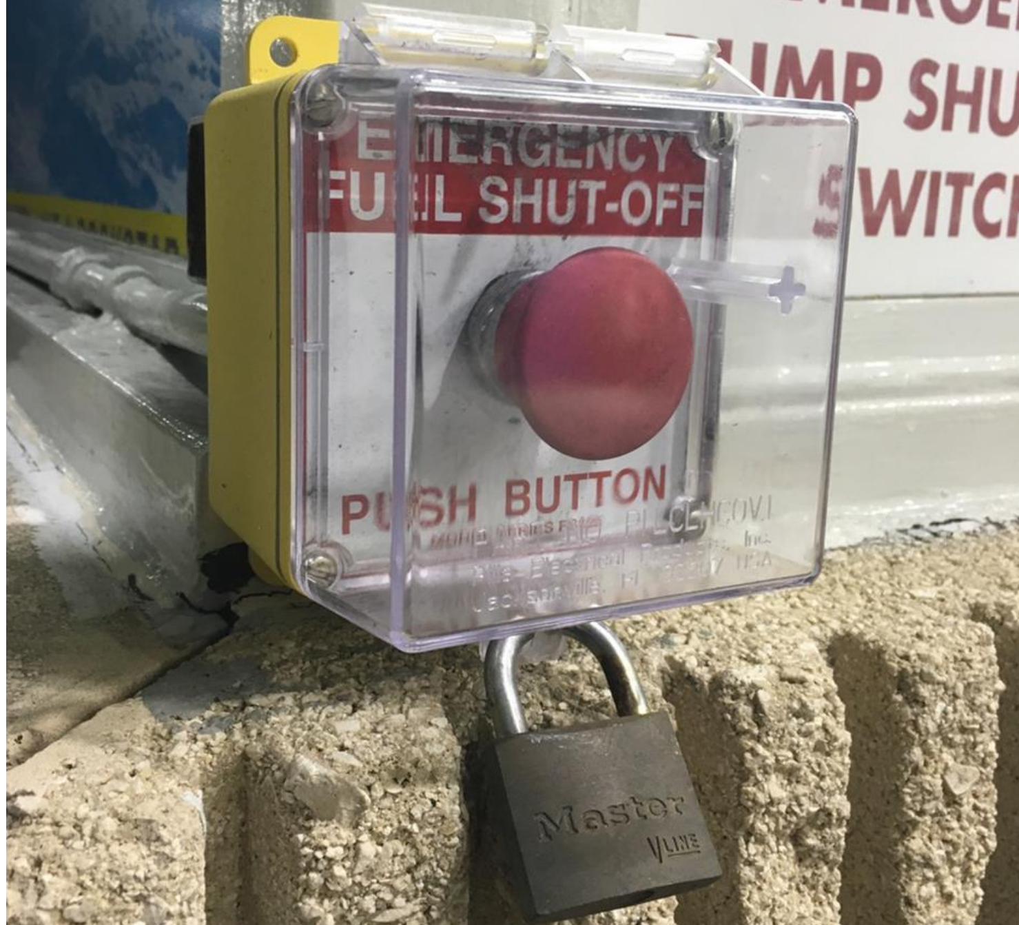
Don't check your fuel level with a lighter at this gas station [Photograph]. (2017). reddit. https://www.reddit.com/r/OSHA/comments/5nbn4t/dont_check_your_fuel_level_with_a_lighter_at_this/?rdt=63657
