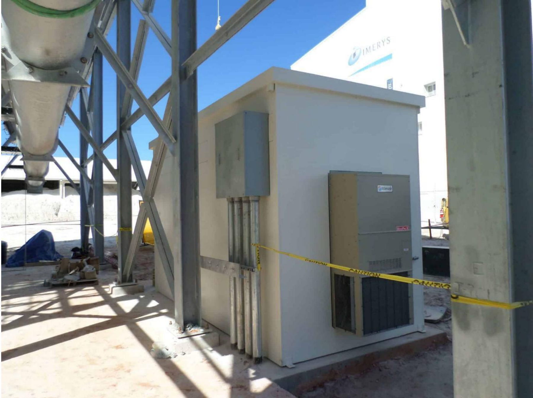
Modular Switchgear Enclosures [Photograph]. (2023, July 19). Porta-King Building Systems. https://www.portaking.com/equipment-enclosures/switchgear-enclosures/
